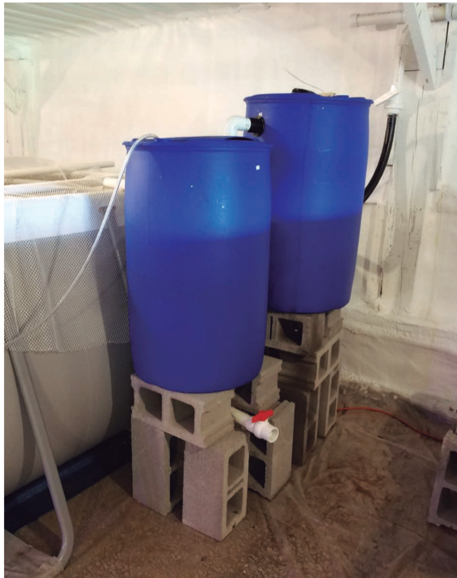
Figure 5. A simple settling chamber and a biofilter. The settling chamber is higher to allow water to travel to the biofilter via gravity. The filters are supported by concrete blocks. Note the protected surfaces in the room and covered tank.
