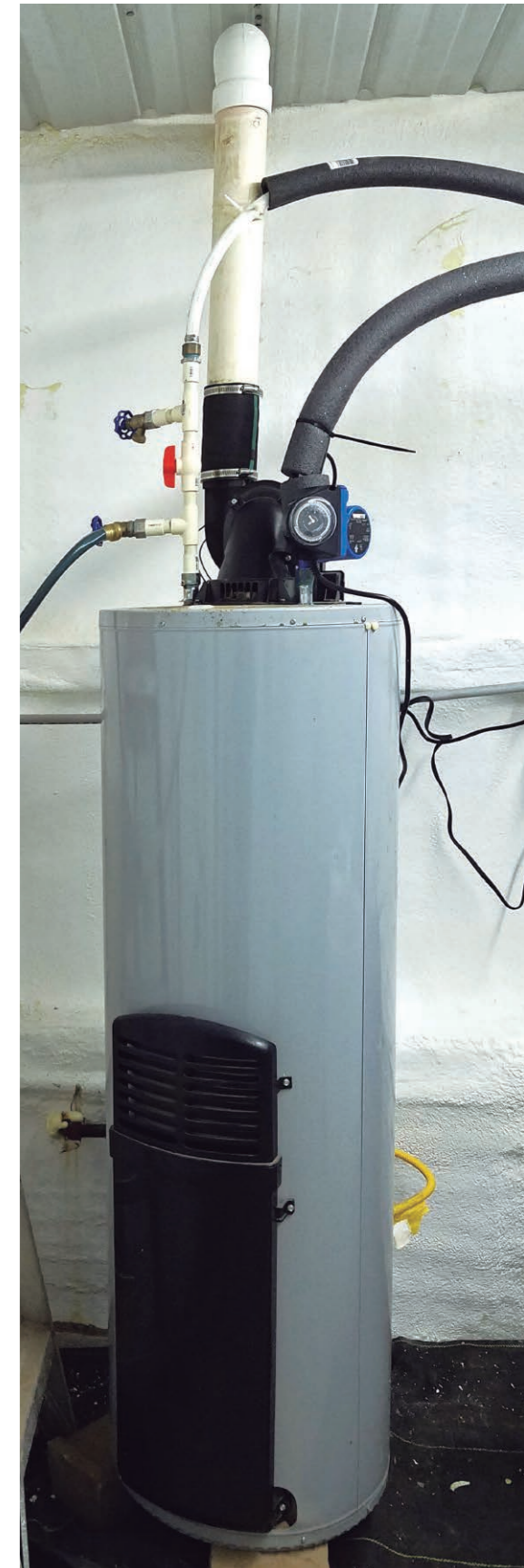
Figure 7. A household water heater with a circulation pump which also has a timer so that it can be operated for a set period of time each day. The water travels to coils of PEX pipe in each shrimp tank, then back to the water heater.
